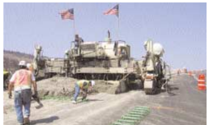
Installing dowel basket “on the fly” in front of paver.
