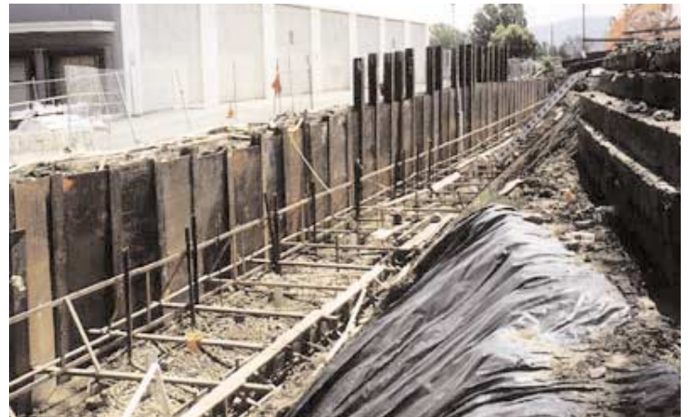
Retaining wall 2 shoring.
