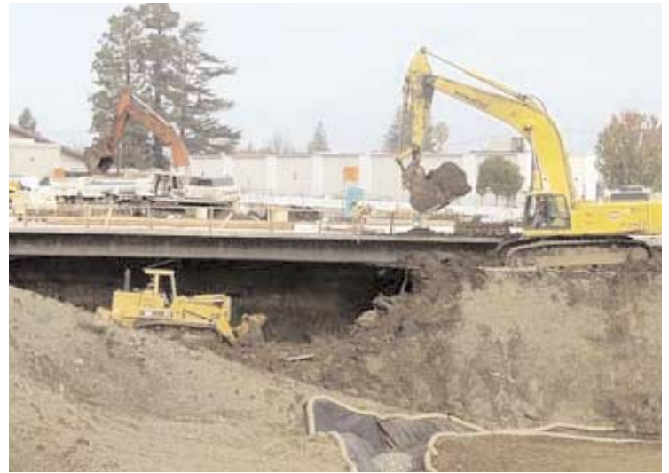
"Mining" after post tensioning.
