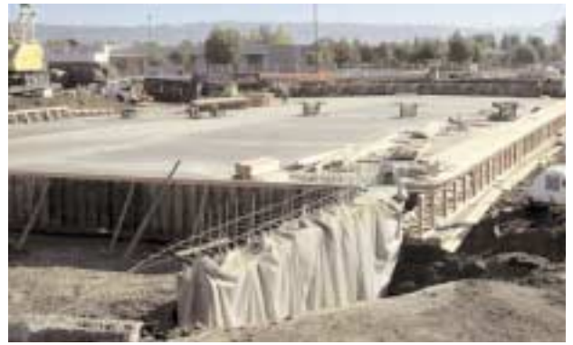
Trancas Bridge on grade construction.
