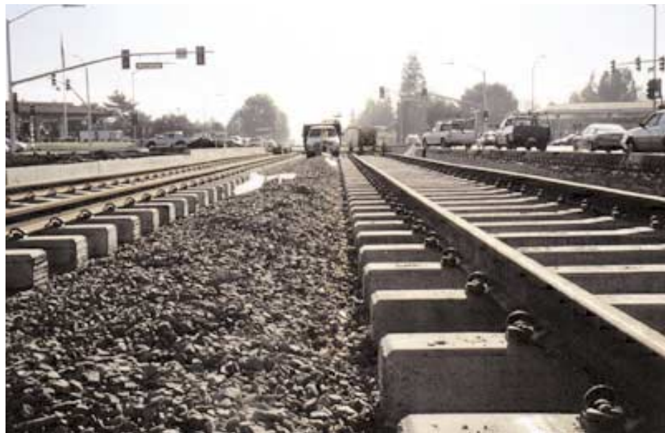
Continuous rail ready for top ballast.
