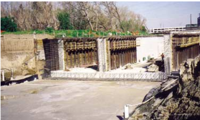
One tie wall forming system.
