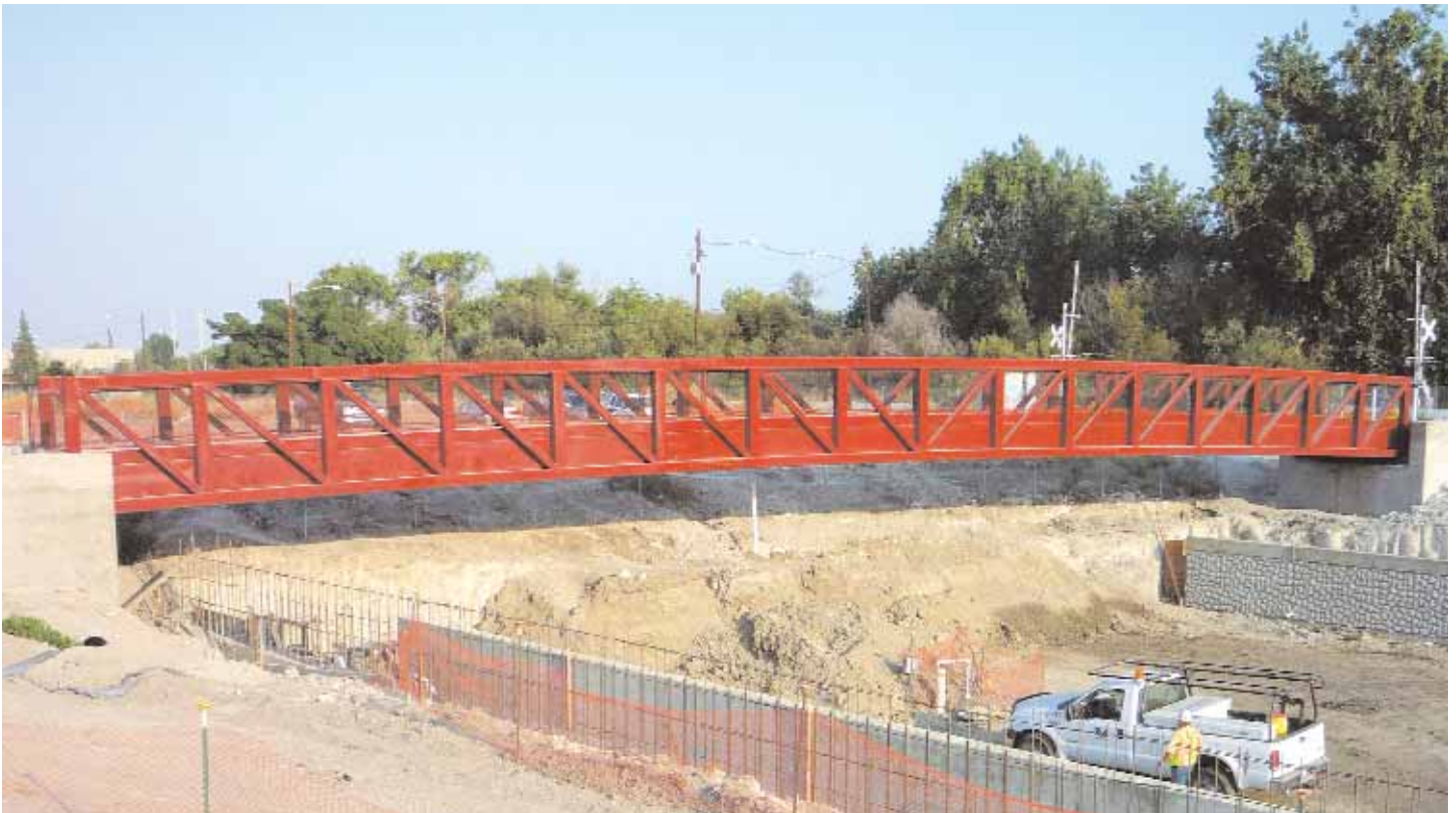
Paseo Padre utility bridge.
