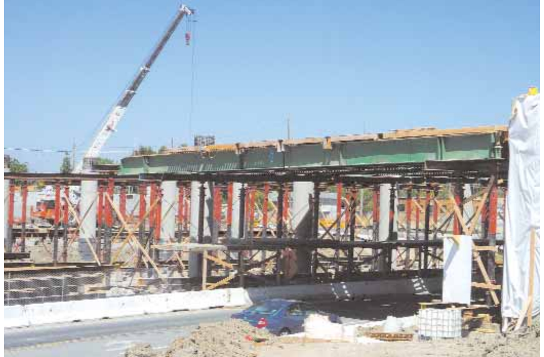
Washington Avenue Bridge falsework installation.
