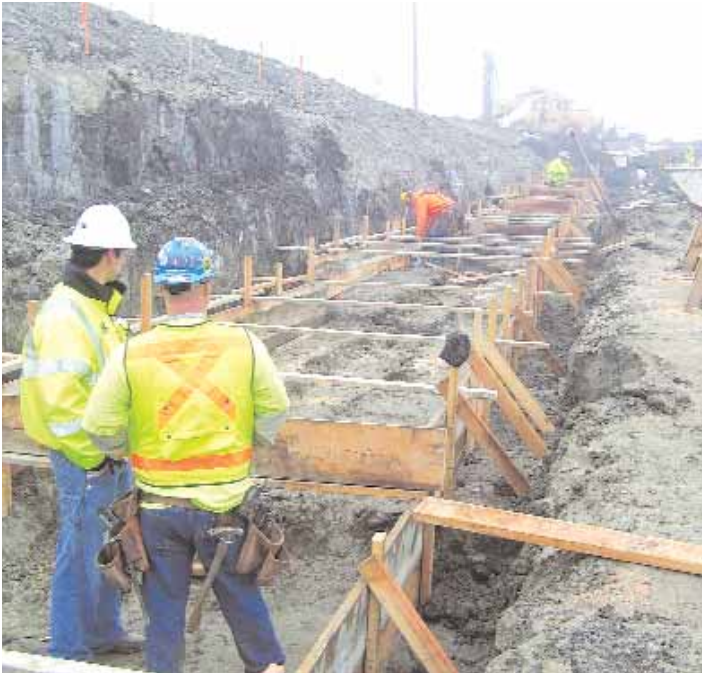
Paseo Padre wall footings.
